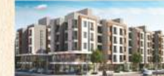
SAMANVAY SPARSH Shops & 2 BHK Apartments @ New Manjalpur
